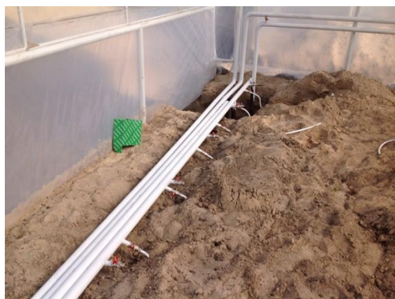
Figure 3. The students could know the methods of greenhouses heating and their disadvantages
